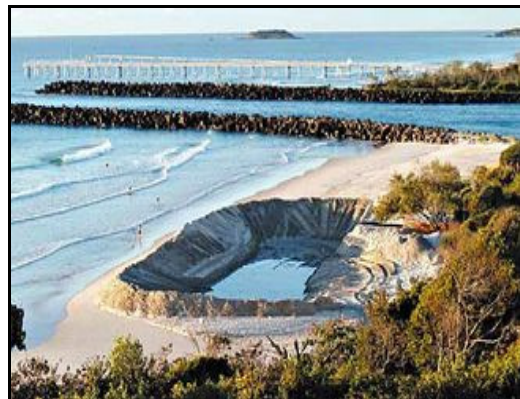
Figure 5 Council bunding works during May 2010 pumping (source: Tweed Daily News)
